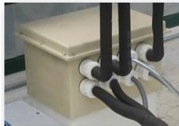
Medium Pipe Chase Housing is designed to accommodate up to 4 split systems (16 lines)
